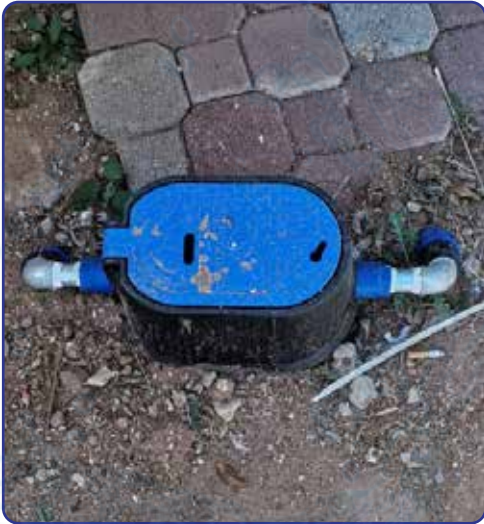
INSTALLED DW109 METERS WITH BOXES IN MOGODITSHANE.
