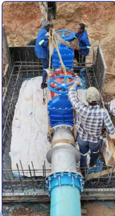
Supply and installation of 400mm Cla-Val Rate of Flow at Rankepa Boatile for W. U. C.
